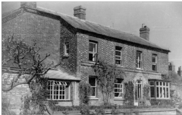
Mill Lane House
